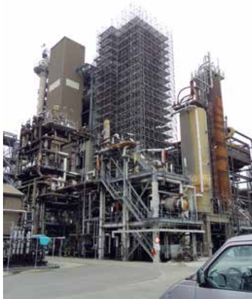
Destillatietoren 2T2001 in de steigers na 3D-scanning.
